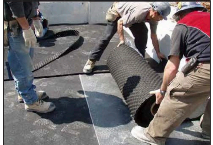
Critical applications use 2 layers ISO-SEP25HD and Perimeter Isolation Board- example: Standby Generators over condo suites.
